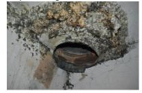
This abandoned exhaust vent provides a direct air leakage path to the exterior. It requires patching.
