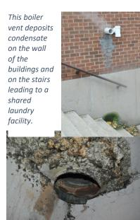
This abandoned exhaust vent provides a direct air leakage path to the exterior. It requires patching.
