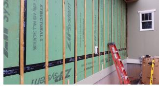
Wood furring strips provide drainage gap (rainscreen)
