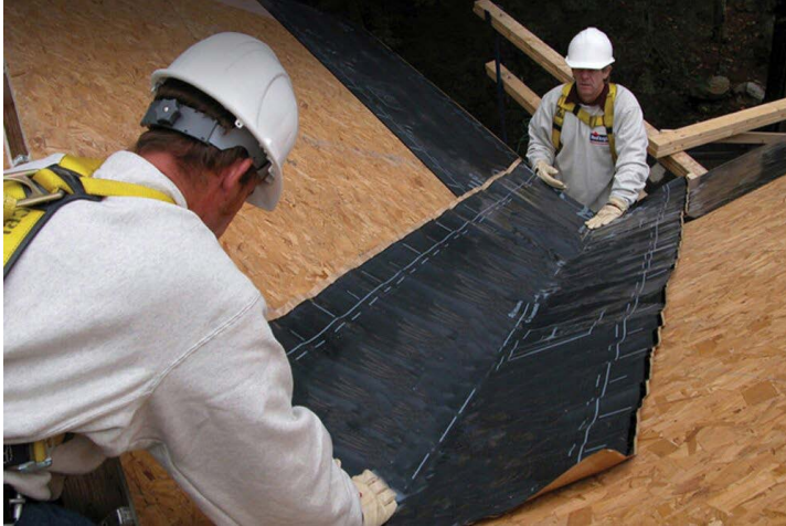
Self-sealing bituminous membrane installed at roof valley
