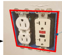
CAULK BETWEEN ELECTRIC BOX AND WALLBOARD
