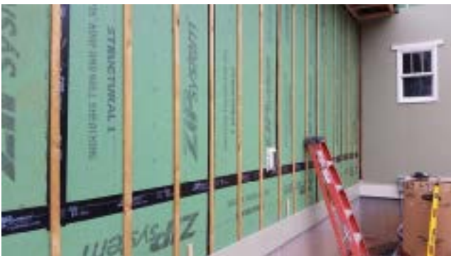
Wood furring strips provide drainage gap (rain-screen)
