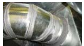
Seal all accessible ductwork.
