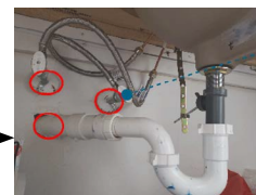
SEAL PIPE PENETRATIONS BELOW SINK
