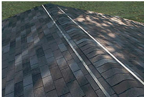
Zinc roof strips, Source: Home Architect
