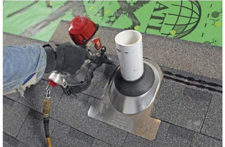
Flashing at roof penetration
