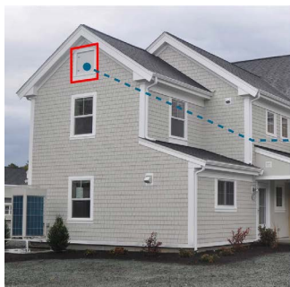
VENTED ATTIC ACCESS THROUGH ROOF GABLE
