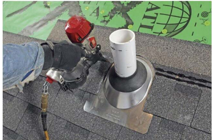
Flashing at roof penetration
