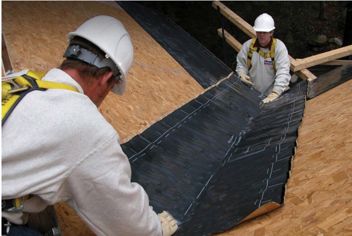
Self-sealing bituminous membrane installed at roof valley
