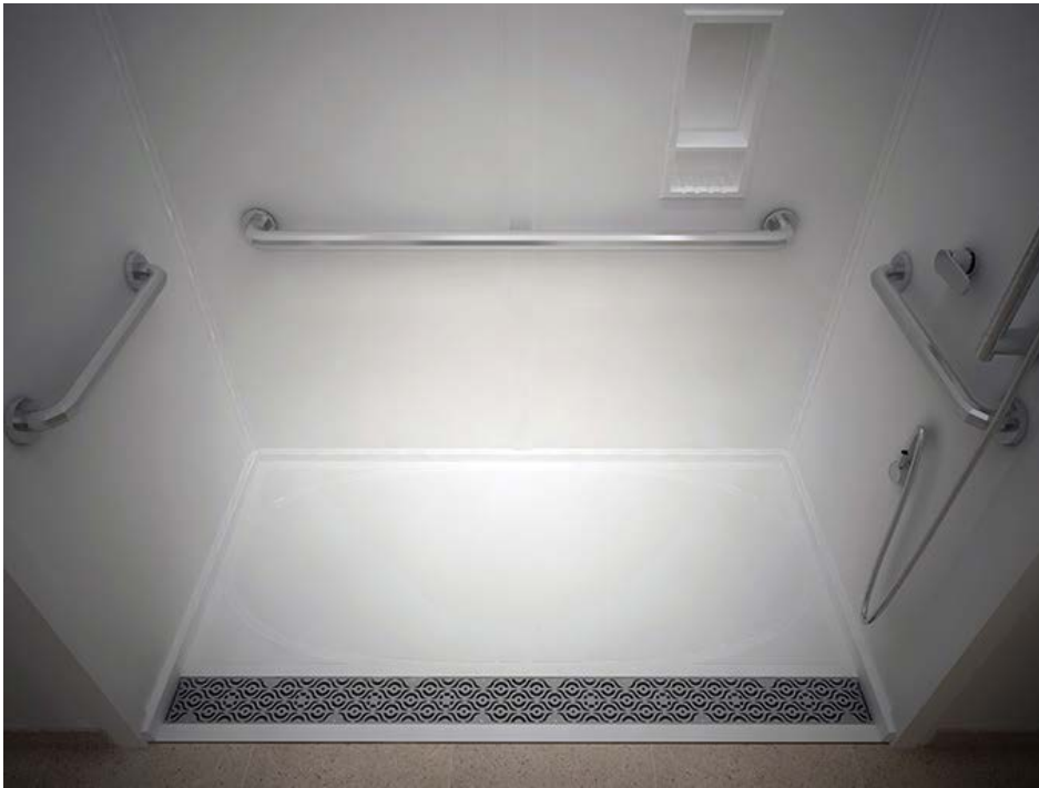
Roll-in shower with trench drain at threshold
