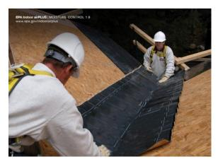
Self-sealing bituminous membrane installed at roof valley
