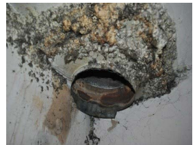
This abandoned exhaust vent provides a direct air leakage path to the exterior. It requires patching.
