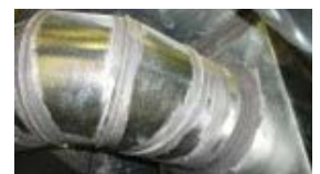
Seal all accessible ductwork.
